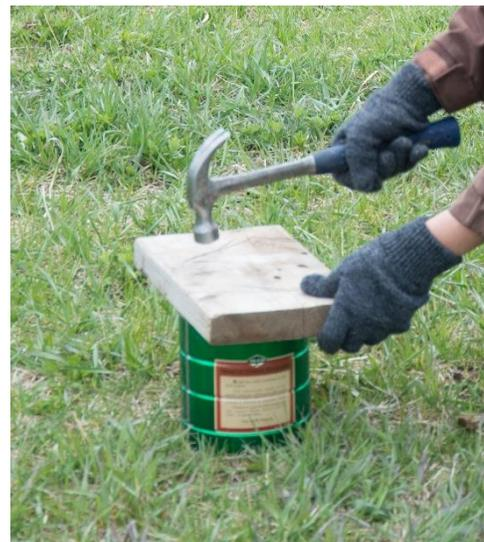
If the soil contains rock fragments and the can cannot be inserted to the appropriate depth, gently push the can into the soil until it hits a rock fragment.
